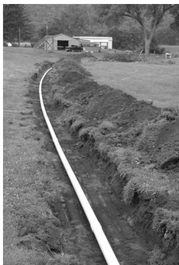
The new pipe snaked it way through the club grounds
