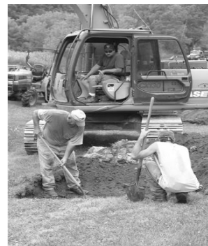
Todd Mathison and Paul Lewison direct Roger Anderson in the digging.
