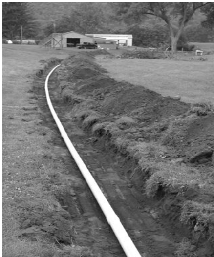
The new pipe snaked it way through the club grounds
