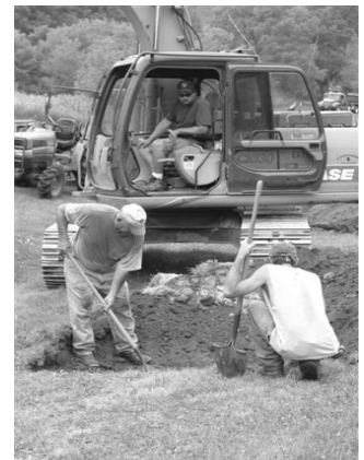
Todd Mathison and Paul Lewison direct Roger Anderson in the digging.
